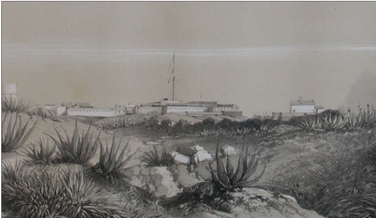
Figure 93: St Helena mast on Ladder Hill (from drawing by Brager, 1840).
