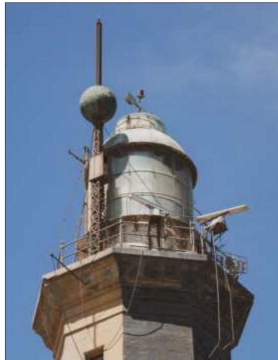
Figure 30: Port Said time ball after decommissioning (copyright, Joel Carillet; reproduced with permission).
