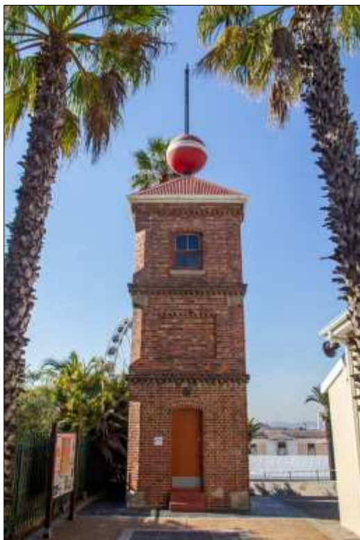
Figure 35: Alfred Docks time ball after restoration (photograph: Michael Peel).
