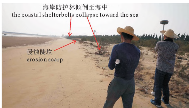
图 6 B 断面南侧的侵蚀现象,海岸防护林倾伏至海中(2017 年) Fig.6 The coast erosion occurred on the south side of section B, caused the coastal shelterbelts to collapse toward the sea(2017 year)
